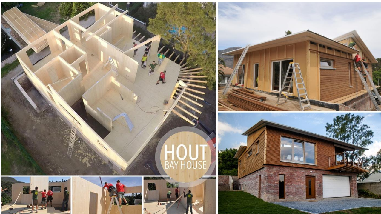
Figure 1: Hout Bay House and its construction
