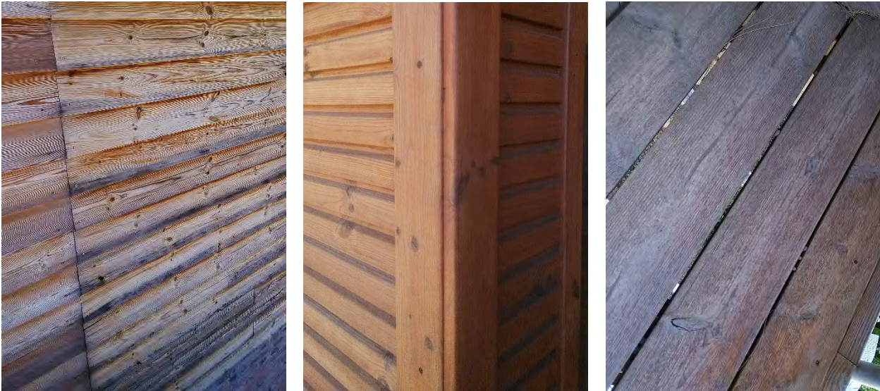
Figure 24: The appearance of wood constructions after 2 years of weathering: untreated facade, treated facade and terrace decking (from left to right)
