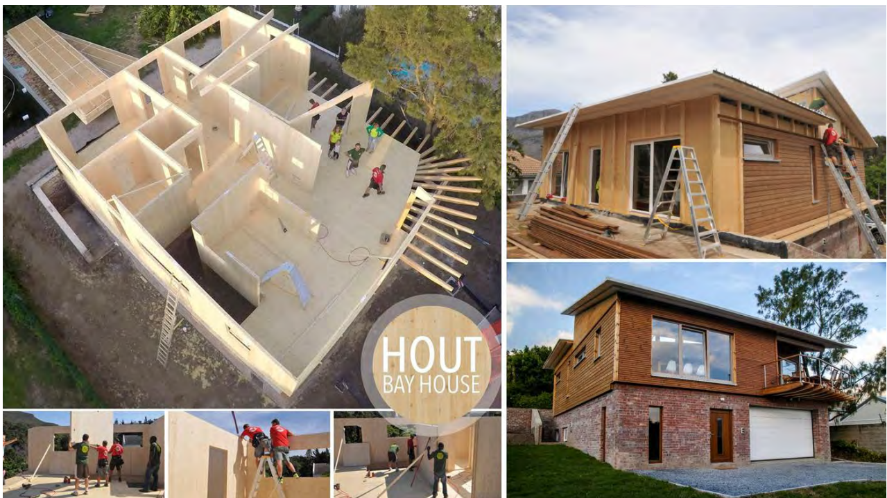
Figure 1: Hout Bay House and its construction
